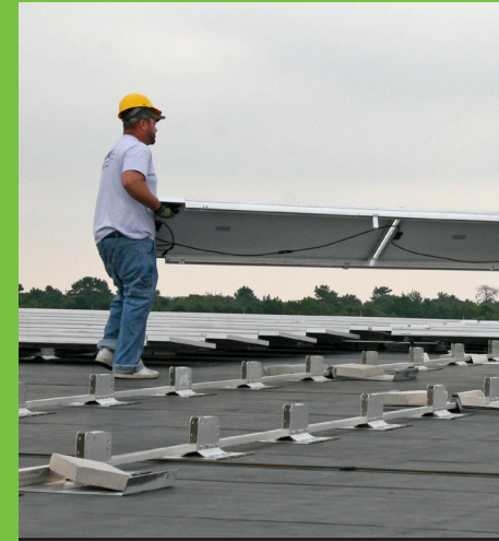
Installing solar panels
